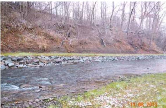
*Looking upstream after construction at rock riprap toe with bench Thomson Cross Road at the top of the bank.*
